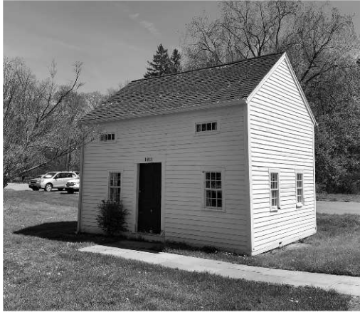
The Captain's House before demolition
